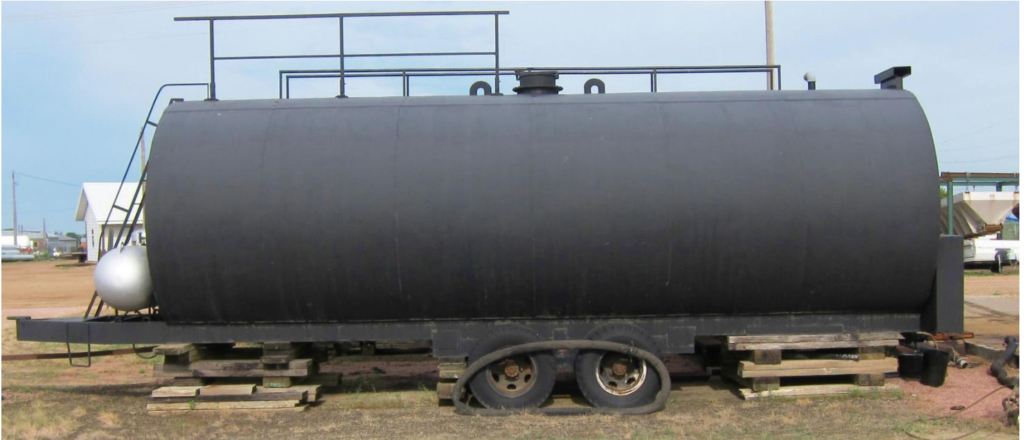
Storage tank before the application of NCI on June 25, 2015.
